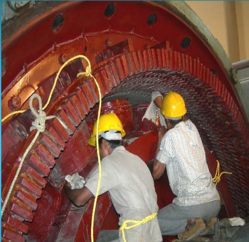
Cleaning the Generator Windings before mounting sensors for retro-fit
